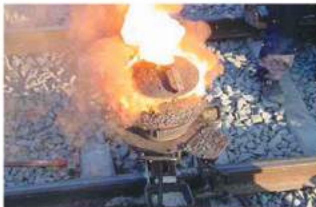
Figure 3-3 Welding of railway with thermite process
