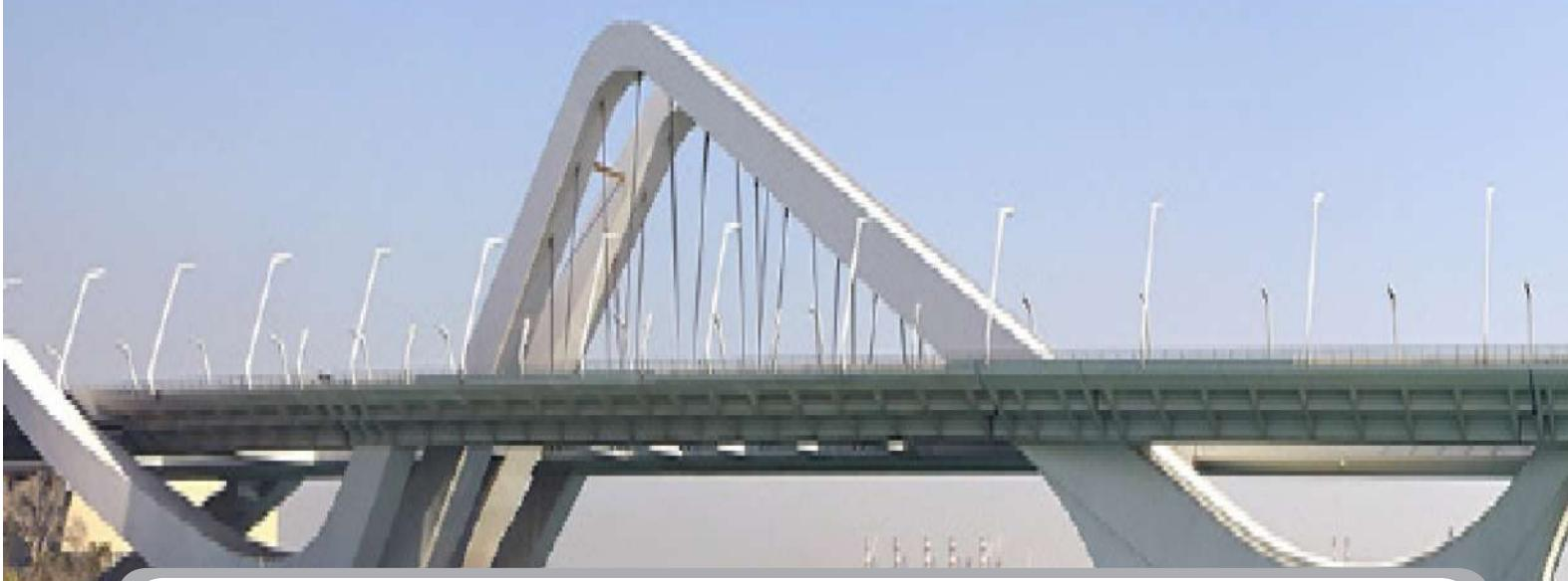
The triangular shapes give the construction strength and firmness, where most of works of the Iraqi architect, the late, Zuhra Hadeed had distinguished by its triangular geometric shapes, one of them a bridge in Abu Dhabi where the height of the triangle top reached to 60m above the sea surface level.
