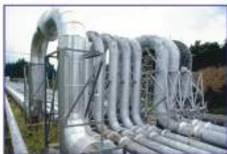
Large bends in pipes
