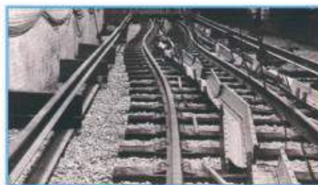
Gaps are placed between railway bars
